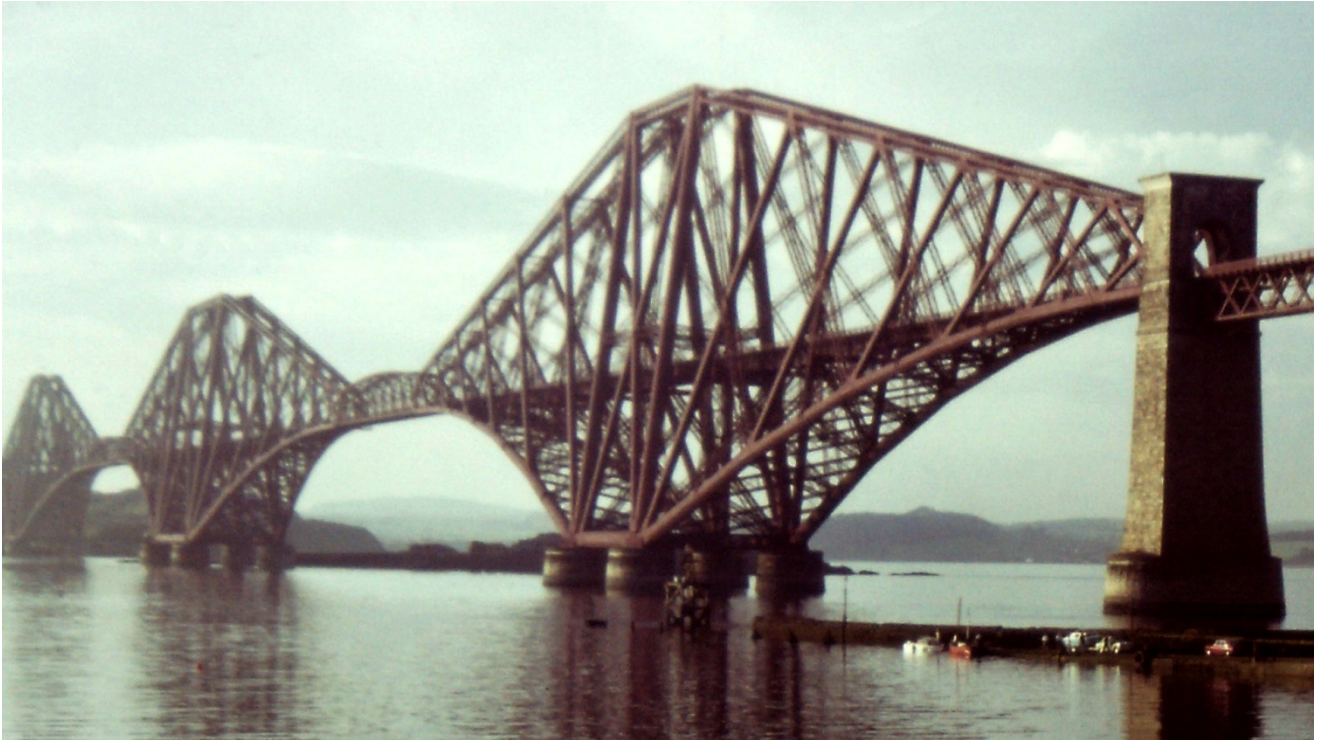
Firth of Forth Bridge by J. Fowler and B. Baker 1889
